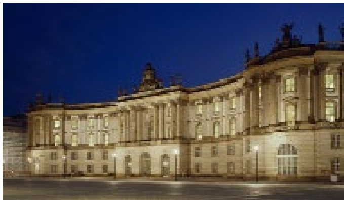
Fig. 75. Floodlight Schröder lighting
